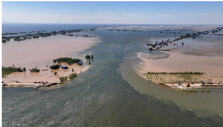
Figure 7. Embankment breach at Tuantzhouyuan, Huarong County, Yueyang, in 2024
